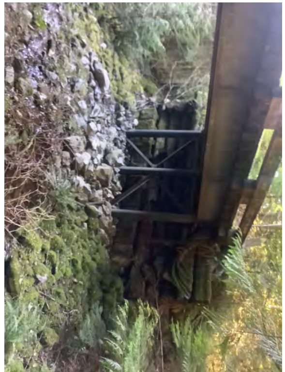
Right Bank Abutment when facing downstream
